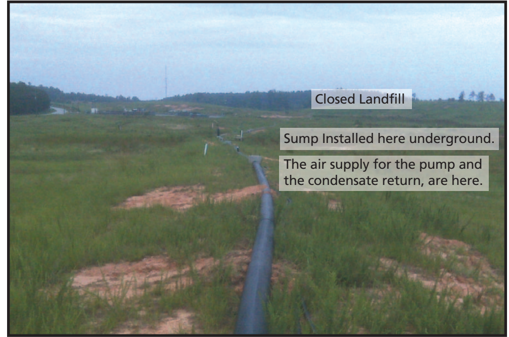
This is an existing pipeline in which a closed landfill is providing methane gas in lieu of natural gas to a neighboring industry.
